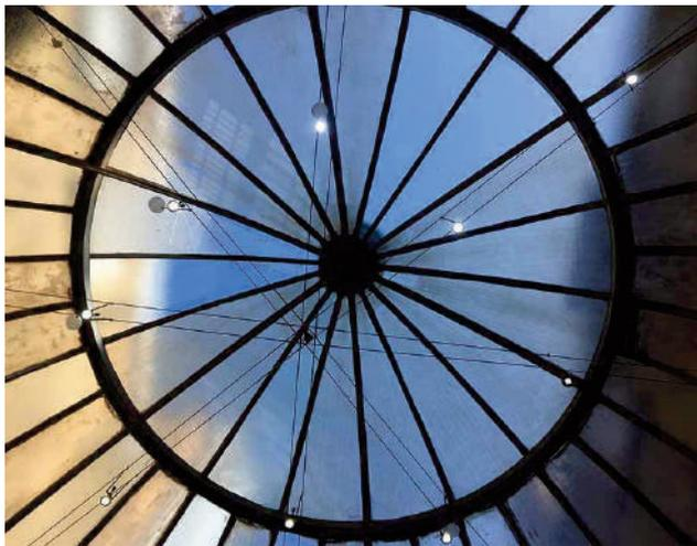
its large and beautiful glass dome which floods the space with light. However, the dome is in urgent need of refurbishment if it is to survive as the structure requires new glazing and refurbishment of the metal framework.
